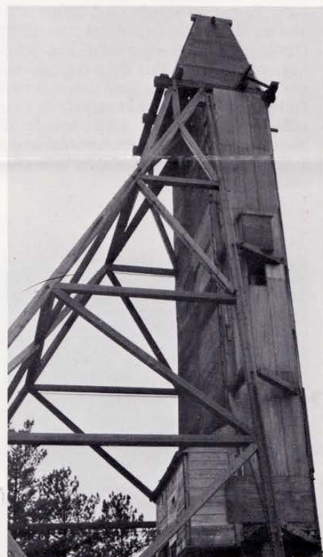
HEADFRAME OF INCO PROPOSED SHAFT SUNK IN 1967.
